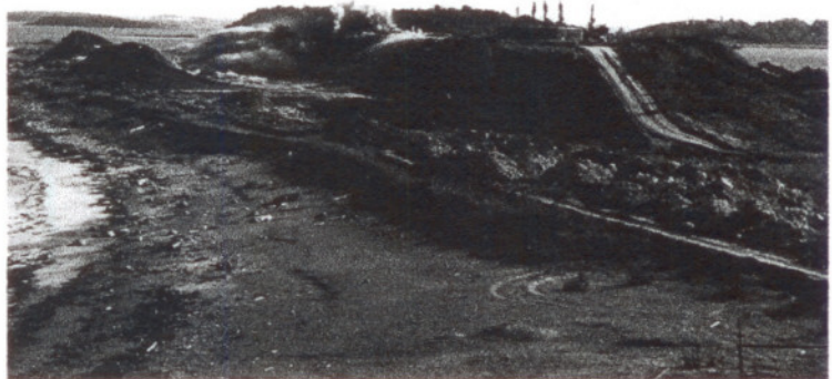
A MILITARY BUNKER IS DEMOLISHED AS PART OF HARBOR PROJECT SITE PREPARATION.
